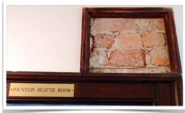
Exposed original door lintel (Photo: Debbie Waugh)
